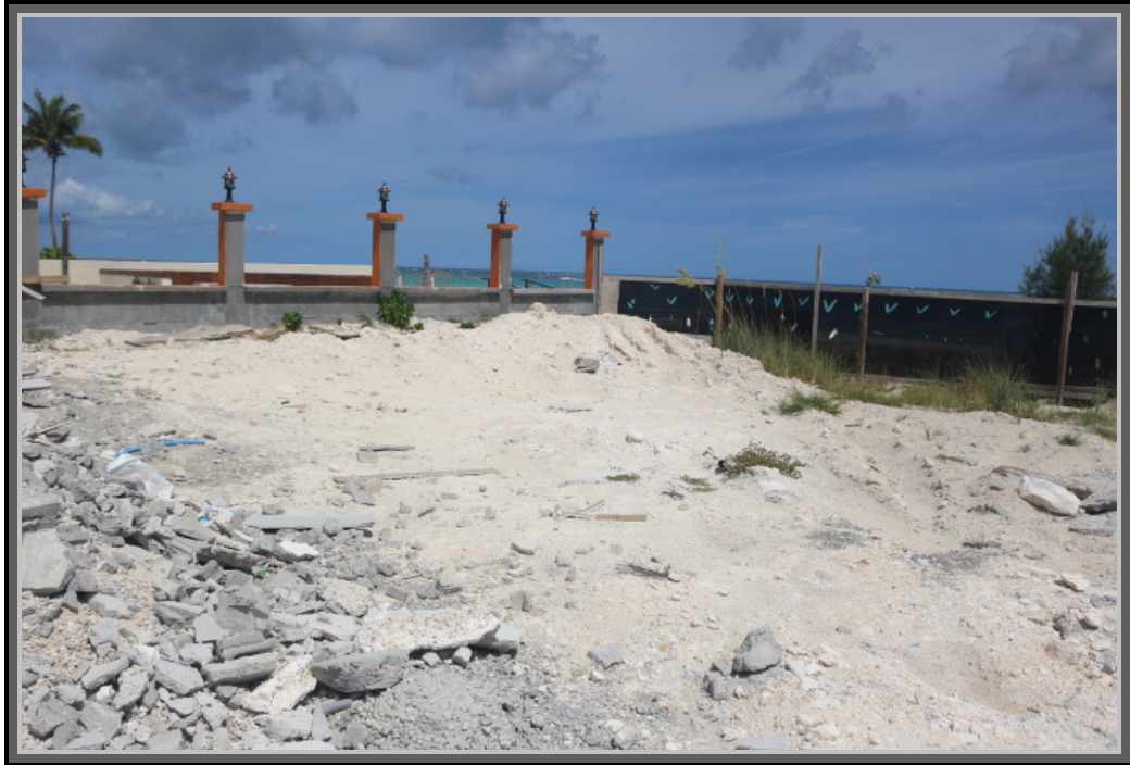
Photo 7.0: Property boundary enclosure. (Date of photo April 14, 2023)
