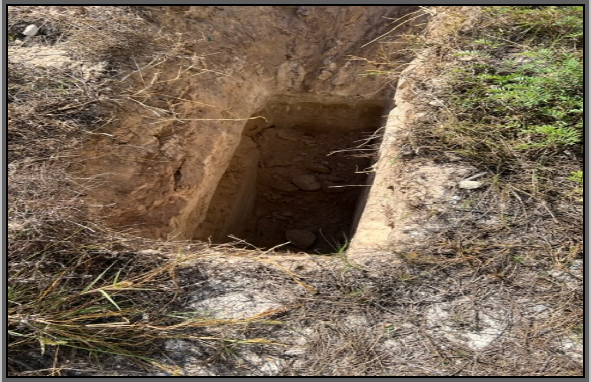
Figure 16.0: Excavated Test Pit
