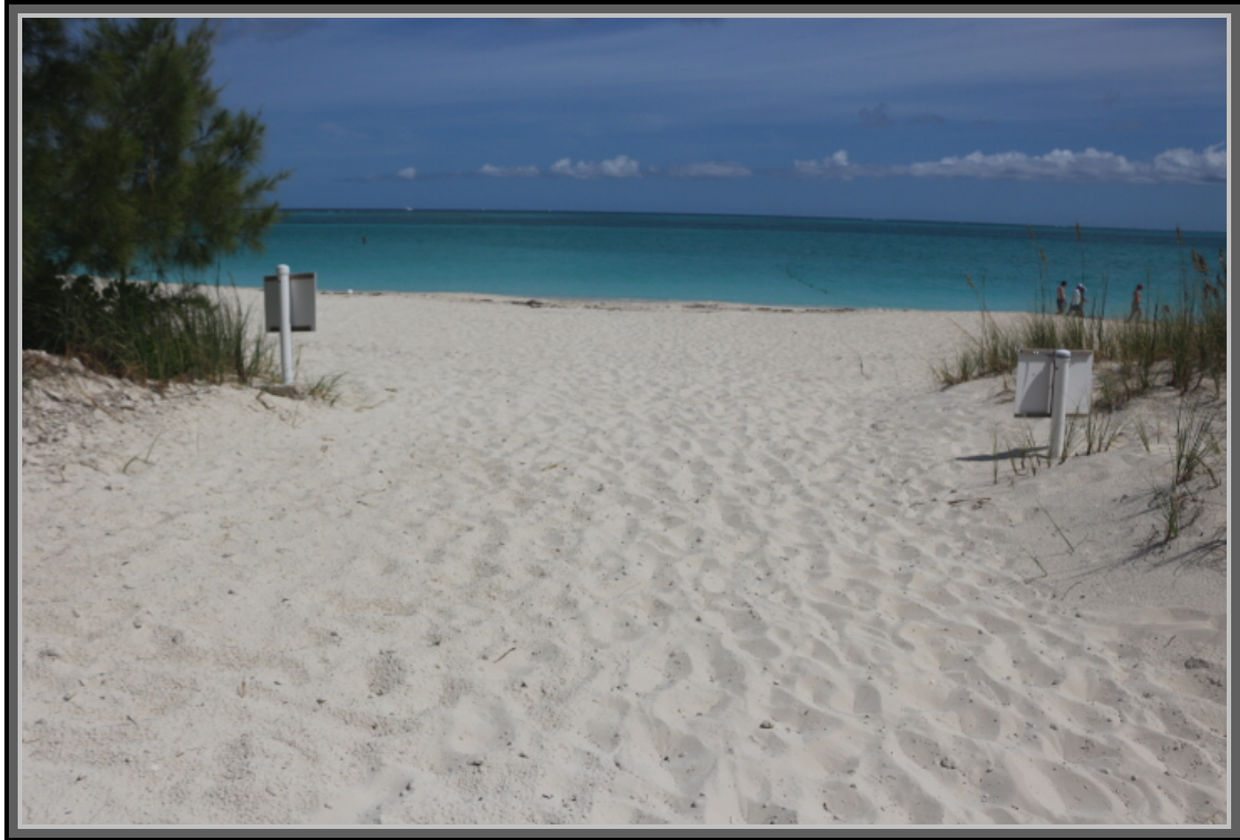
Photo 10.0: Damaged sand dune system to be restored. (Date of photo April 14, 2023)
