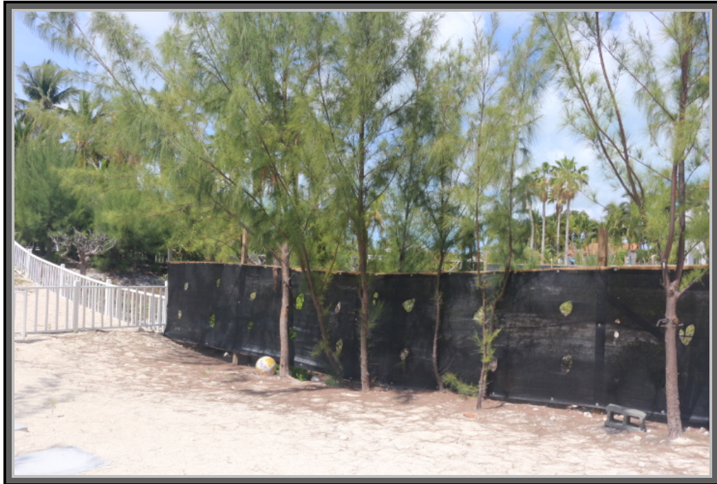
Photo 45.O: Hoarding and screening of construction site
