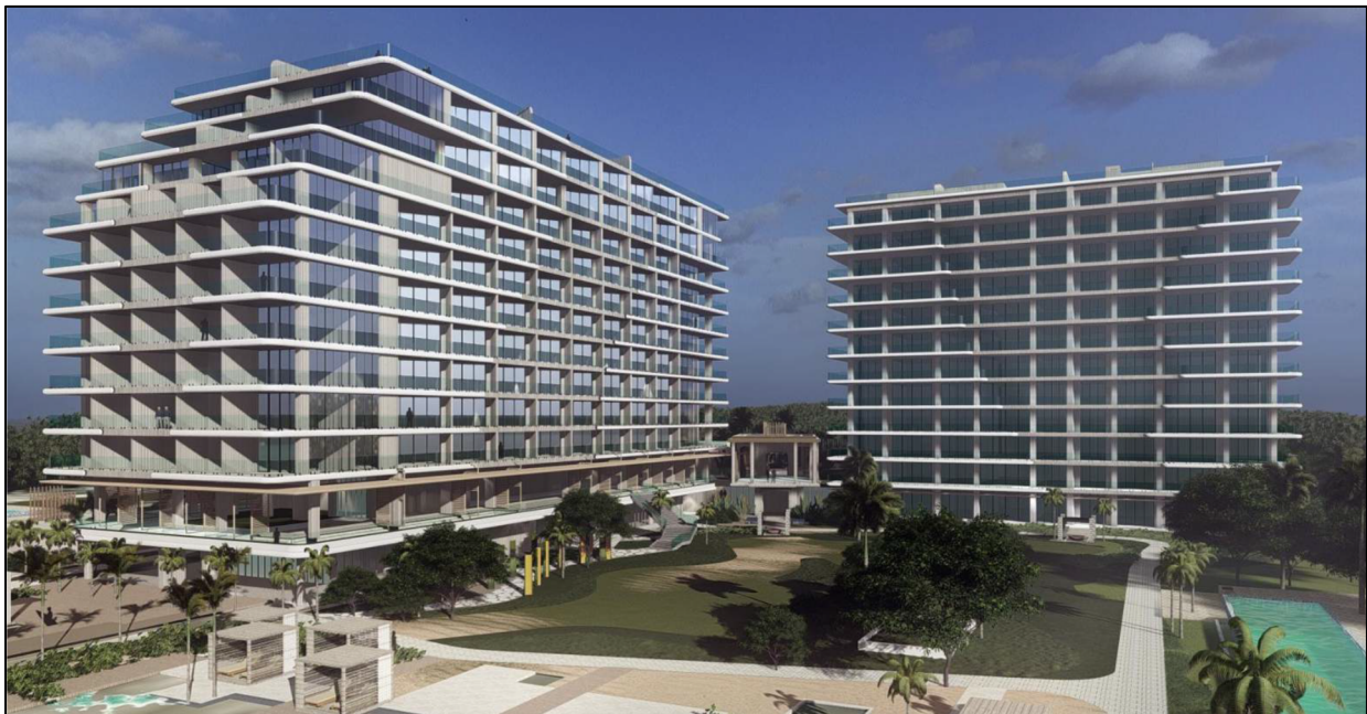
Figure 3-4 Hotel and Residences Pool and Beach Access
